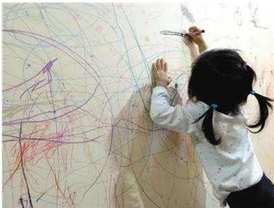
Damaged walls are the most common required repairs before departure
